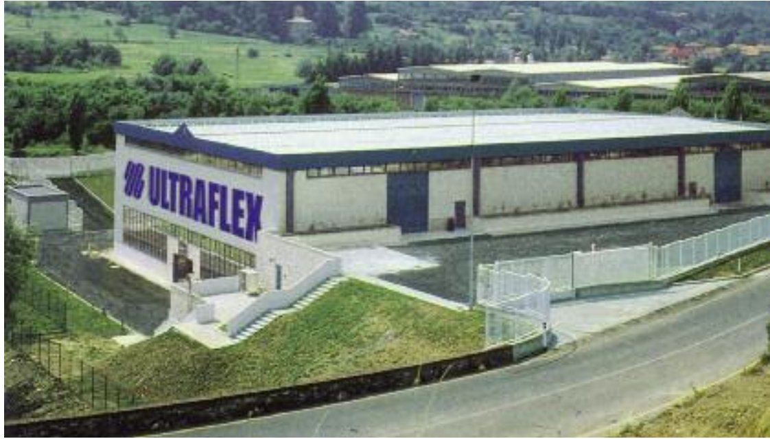
ULTRAFLEX - Factory in Casella
